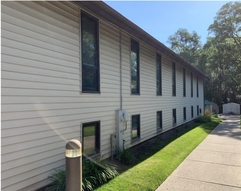
Figure 2a – Daycare center, South Perimeter
