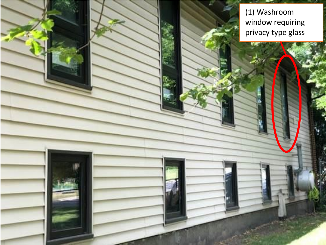
Figure 3 – Daycare center, North Perimeter
