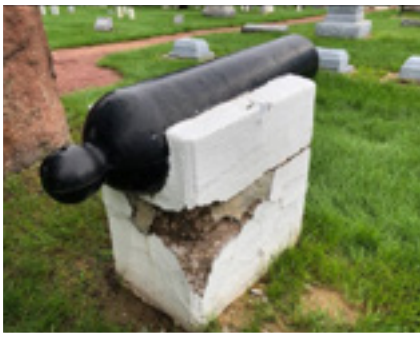
CANNON IN DISREPAIR
